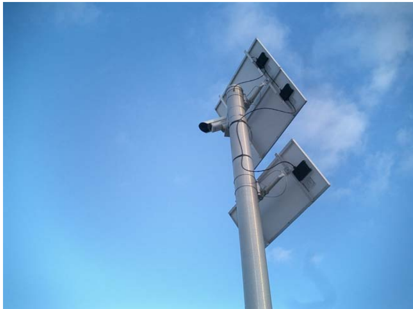
Optical Camera mounted approximately 30' above road surface. Camera installed behind Solar Panels.
